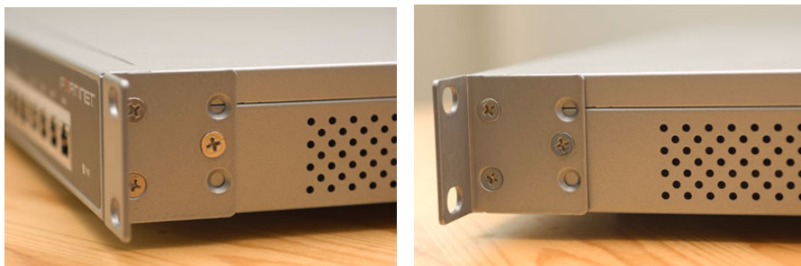
Figure 2: Installed mounting brackets
